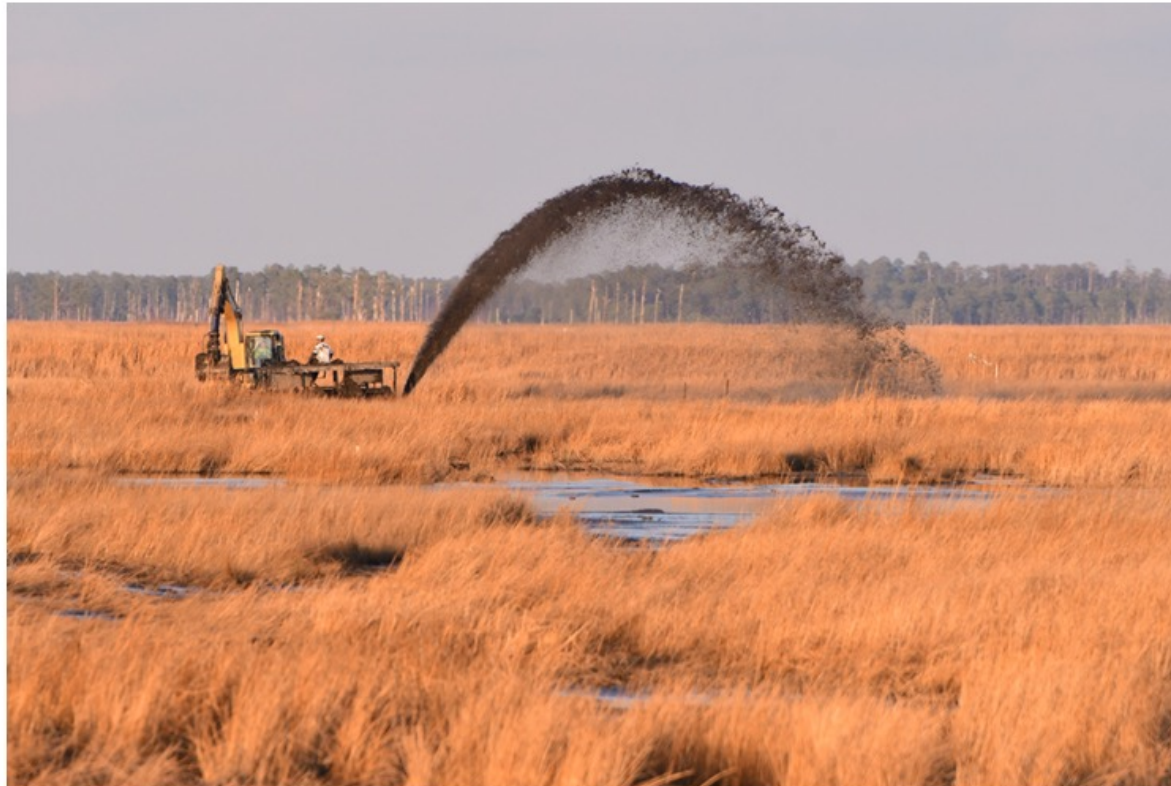
Building up a portion of marsh at Blackwater National Wildlife Refuge with sediment from the Blackwater River. (Photo: Middleton Evans)
