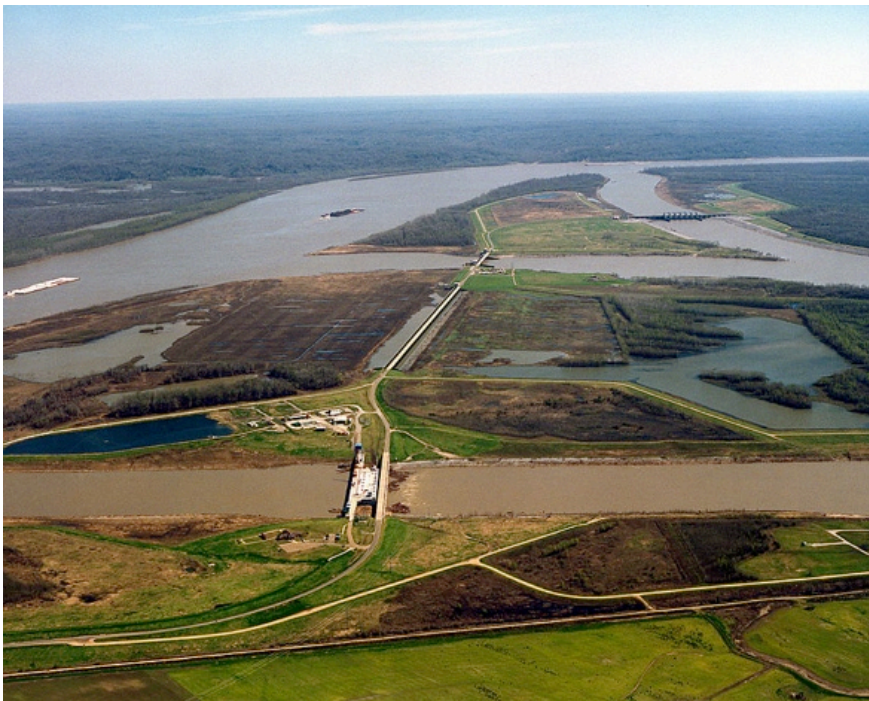
Old River Control Structure
